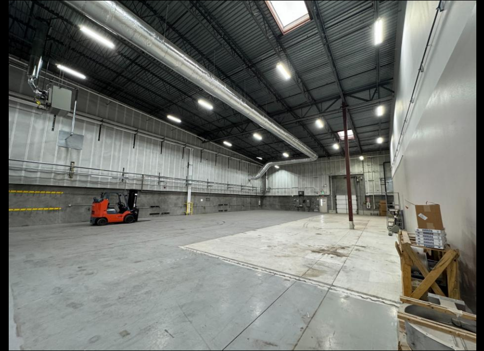
FusionWERX will operate under a broad-scope radioactive materials license with most advanced tritium handling capacities available in the private sector when fully licensed and operational.
