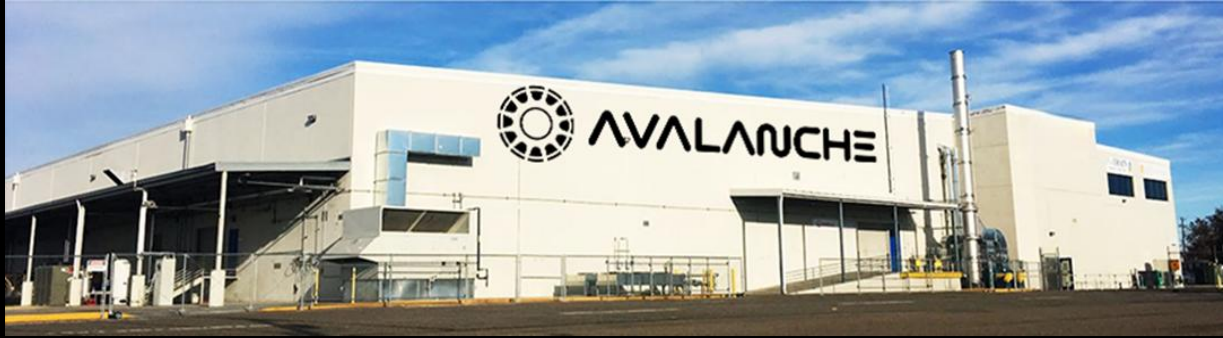
FusionWERX in Richland, WA, USA is a first-of-its-kind commercial-scale testing facility for advanced fusion technologies
