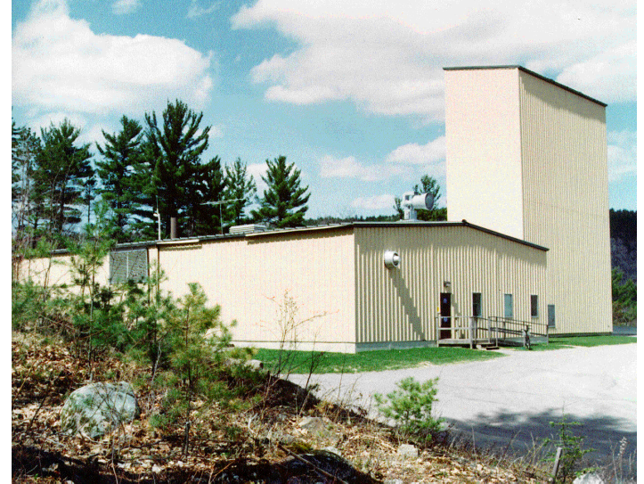
CECE Demonstration Plant at Chalk River Laboratories
